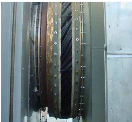
Ø89 inch diameter Gas Turbine Exhaust Expansion Joint with Hot to Cold Frame. 25 in wc at 980°F.
