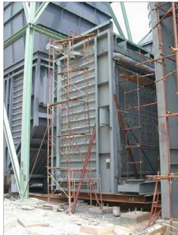
Conversion of simple cycle elbow to fully functional diverter for an Alstom GT13E2 in Viet Nam
