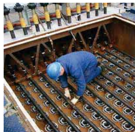
Bag filter maintenance
