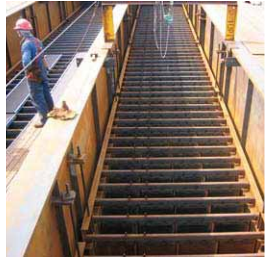
Installation of replacement ESP internals
