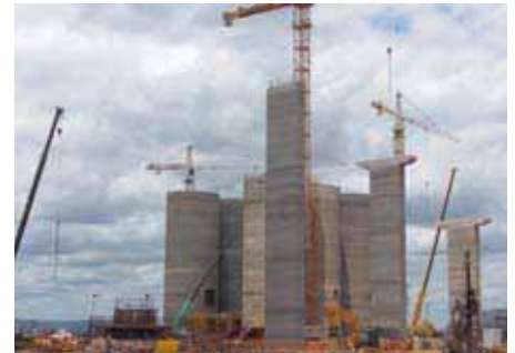
Fly ash silos under construction
