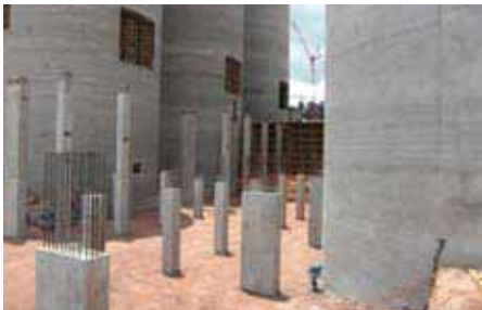
Preparation of one section for the fly ash conveying systems
