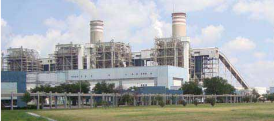
Comision Federal de Electricidad's Carbon II Power Plant in Mexico
