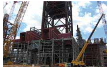
Duct work under construction
