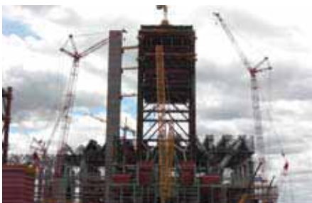
The first out of six supercritical 800 MW boilers under construction
