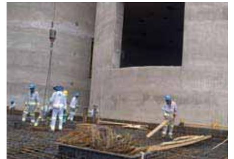
Construction work at the conditioner building
