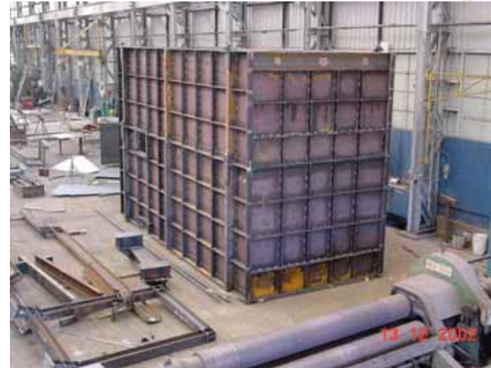
Trial Assembly of Casings prior to paint
