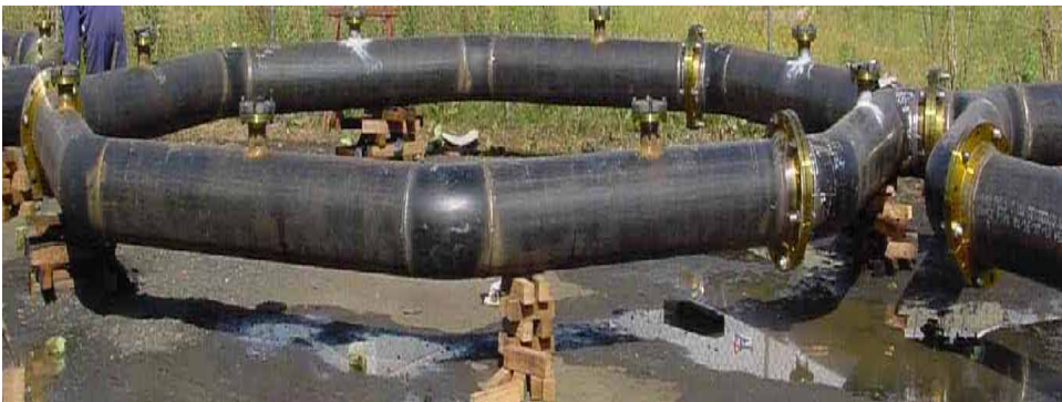
Hydro Testing Ring Main
